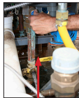
Relief valve - check operation and open to drain unit
