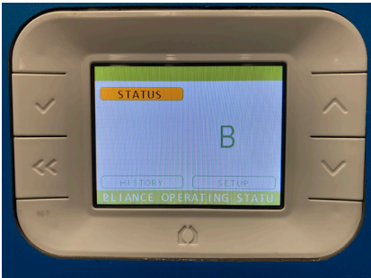
BDB—Boiler Display Board
